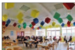
Panneaux absorbants – © Acoustissimo
