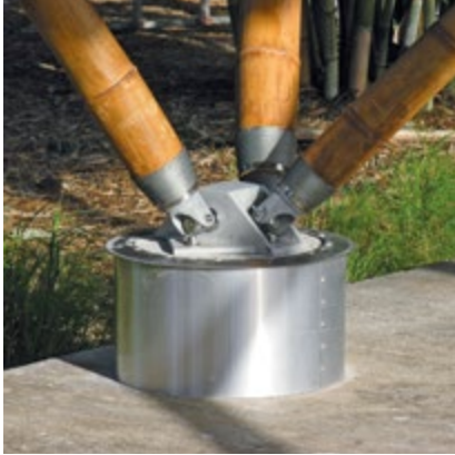
Principe d'attache GUADUATECH – www.guaduatech.com
