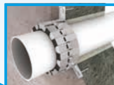
fire stopping et fire sealing
